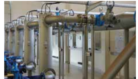
INSTALLED BARRIER S UNITS
